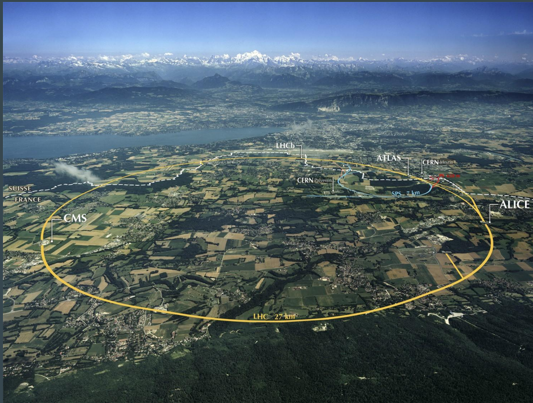
Underground 27 km tunnel
